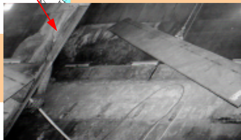
Stainless Steel Cricket Being Added To Existing Wet-Bottom Ash Hopper
