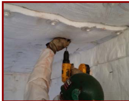
CERABOLTS are easily installed with a cordless power drill and an 11/16" (17mm) socket.
